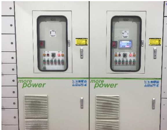
Figure 5 The Merus™ HPQ solution installation
