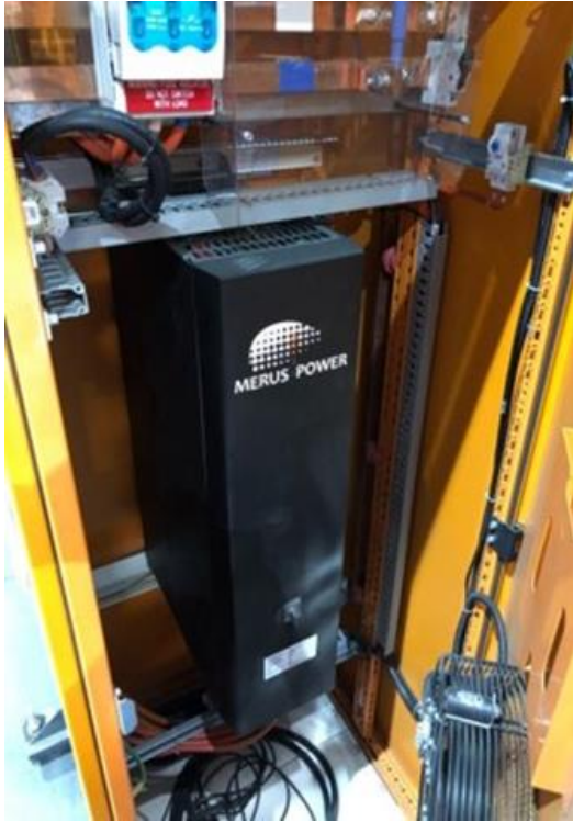
Figure 5 AHF 400 V 50 Hz 100 A at site
